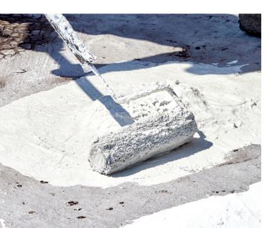
Enduris Bitumen Bleed Blocker is part of the complete Enduris Roof Coating system. Applied as a base coat to asphaltic and bitumenous substrates and surfaces, it is formulated to seal out oils that can discolor the finished coat, helping to protect your investment.
